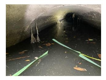
Pipe ID **E15\_D16** is a 30" reinforced concrete pipe with a flared end section. The outfall drains surface water from parts of Arboretum Drive, Deer Island Lane and Moreland Drive. The pipe holds very little water and is free and clear of any obstructions. Picture below is taken at the pipe outlet into Landfall Lake.
