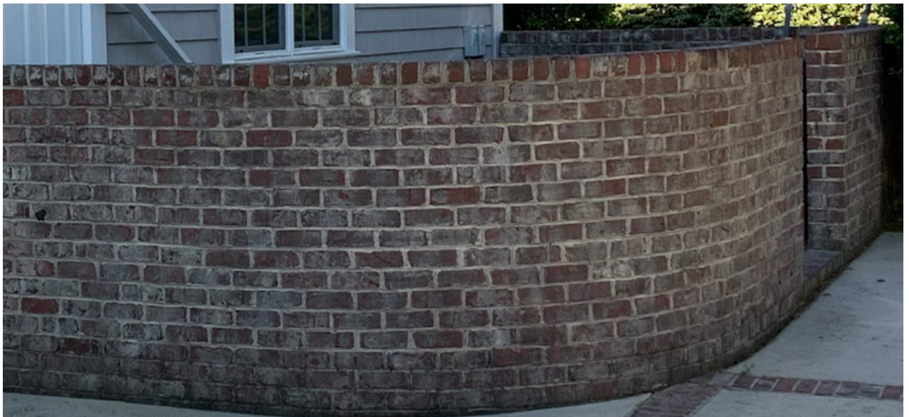
Brick walls - to match existing brick (photo is existing equipment walls)
