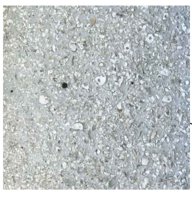
Bench Seat and Planter Foundation, Pool Wall Facade and Storage Enclosure Exterior: Tabby Shell Finish
